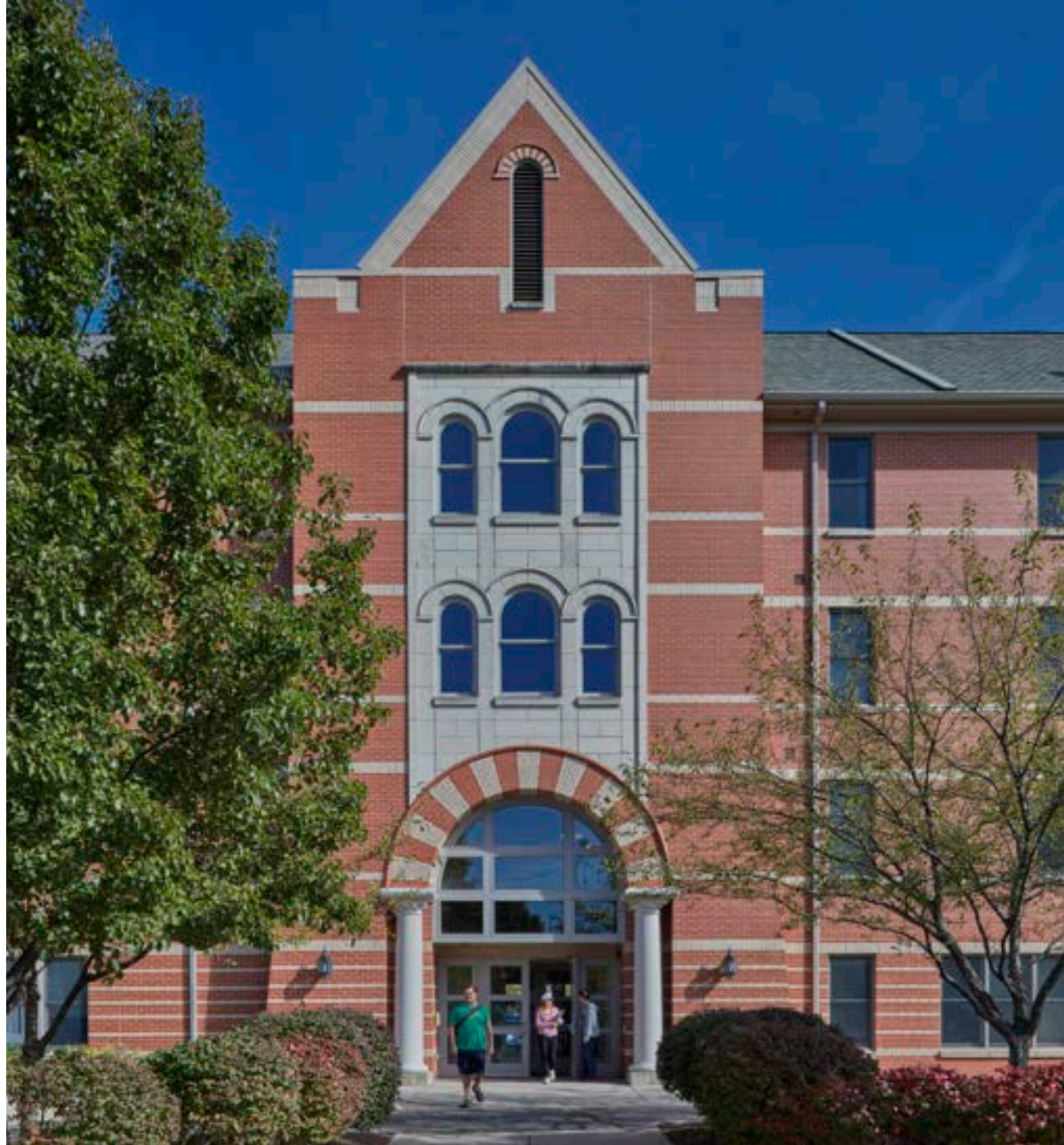
Existing Winter Hall
