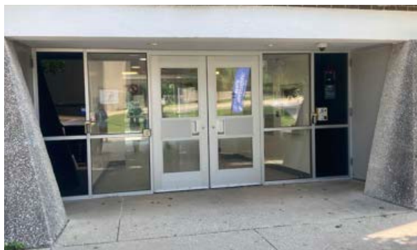
Existing Conditions: Copeland Living Center
